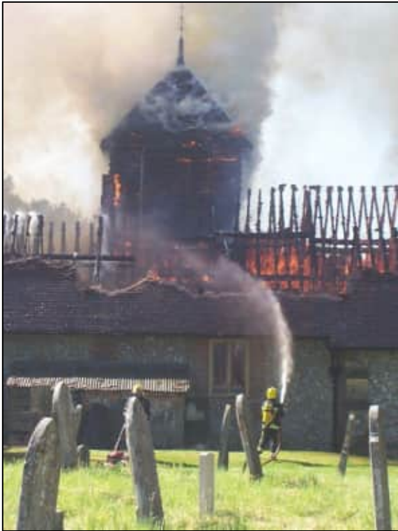
The tower in flames, with the rest of the church gutted
