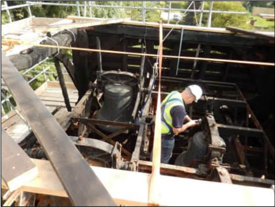
A workman wearing a safety harness carefully releases one of the bells
