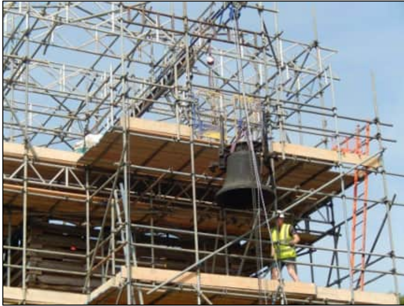
One of the bells is carefully lowered through the scaffolding
